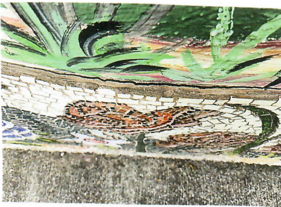
Cracks in Tile work 100+ old Schools Foundation is settling
