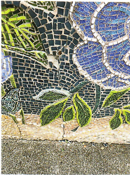
Cracks in Tile work 100+ old Schools Foundation is settling
