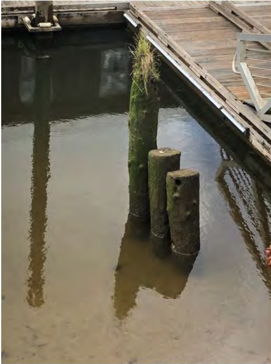
Photo 1: View to the west showing the three piles to be removed as mitigation.
