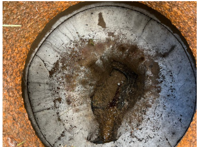
Manhole: H-26 Depth: 4ft
