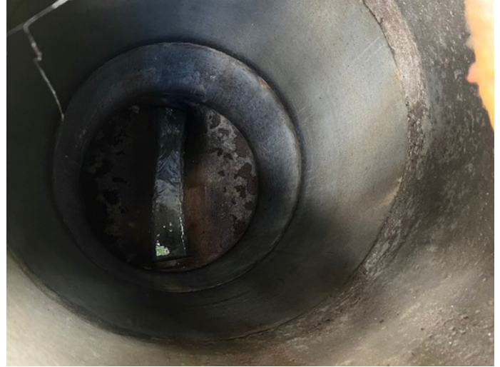
Manhole: H-33 Depth: 10ft
