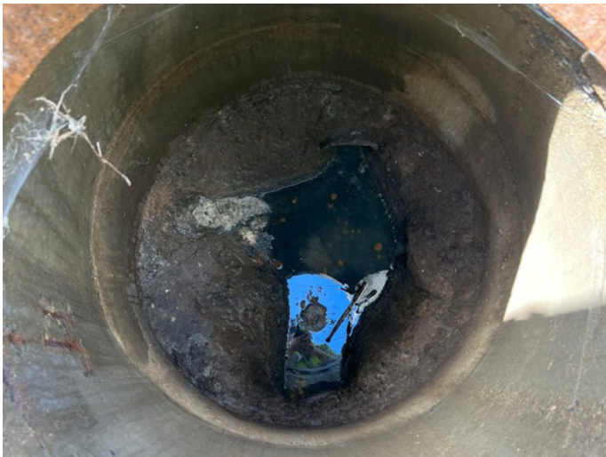
Manhole: K-33 Depth: 6ft
