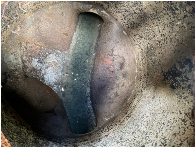
Manhole: H-32 Depth: 3ft
