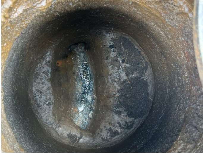
Manhole: B-78A Depth: 5ft
