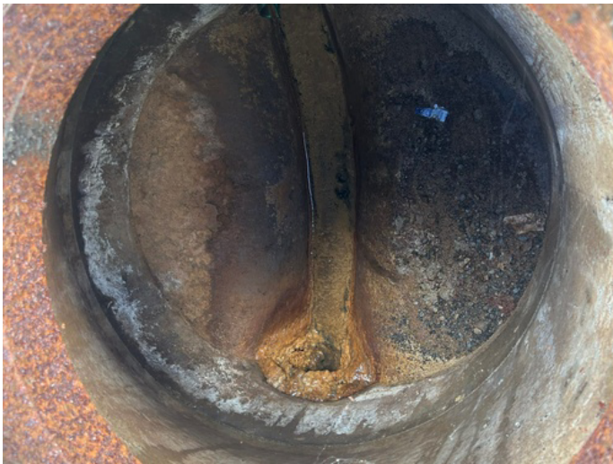
Manhole: J-3 Depth: 5ft
