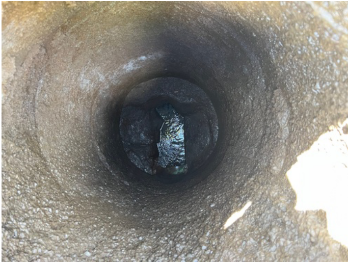
Manhole: K-7 Depth: 10ft
