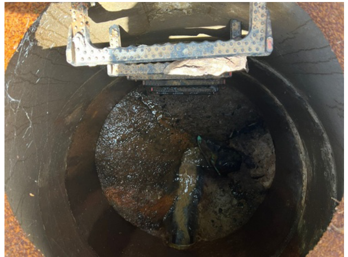
Manhole: E-1 Depth: 7ft
