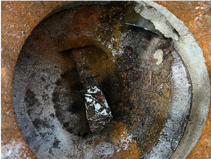
Manhole: H-27 Depth: 4ft
