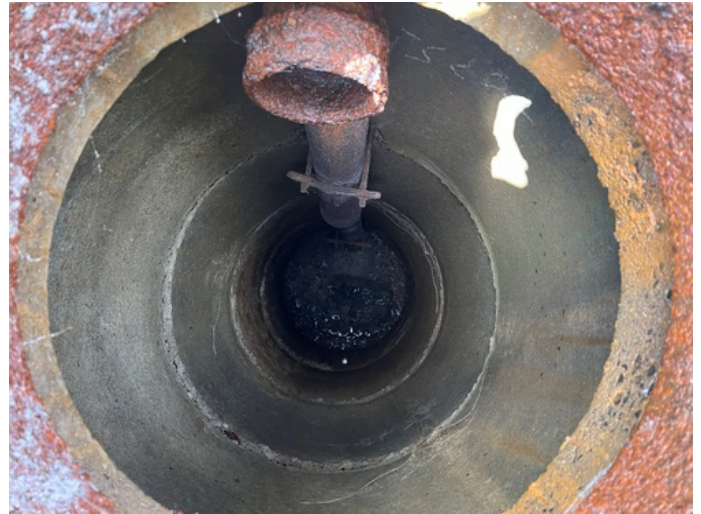
Manhole: K-35 Depth: 15ft
